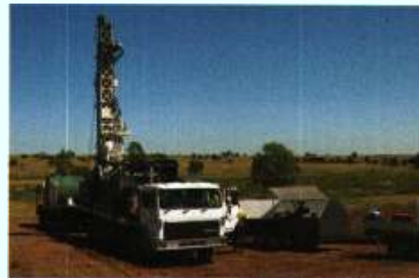
Drilling is underway near Wandoan
