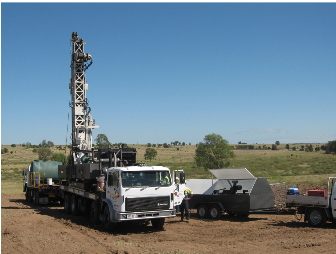
Drilling on MetroCoal's Surat UCG coal project – March
